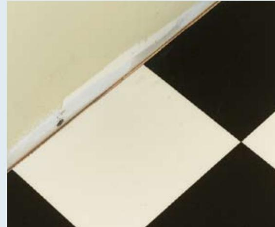
**Leave gaps.** To allow for the normal movement and expansion of the floor and wall surfaces, the flooring must be cut  $\frac{3}{16}$ " to  $\frac{1}{4}$ " away from all vertical surfaces such as walls, cabinets, or pipes. Use a jamb saw to undercut door trim—this will allow for expansion. Make sure vinyl is not contacting the wall surface behind the door trim. Check the fit of the no-glue flooring and then carefully remove the flooring.
