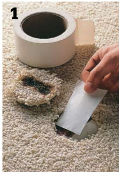
**1 Remove extensive damage** or stains with a "cookie-cutter" tool, available at carpeting stores. Press the cutter down over the damaged area and twist it to cut away the carpet.
