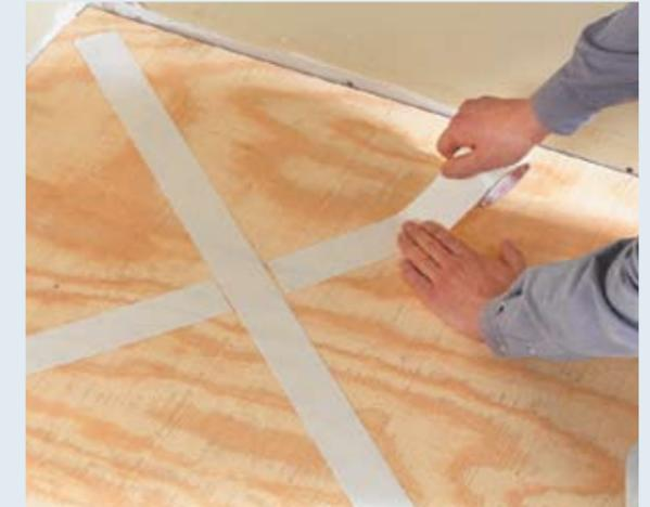
**Place acrylic double-face tape** in areas that will be under heavy appliances such as stoves and refrigerators. Make an X with three pieces of tape—one long piece and two short pieces—so that the tape does not overlap. Place acrylic double-face tape at doorways and under seam lines. Leave the paper covering in place and press the tape down so it adheres well to the subfloor.
