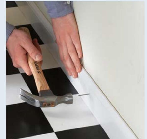
**Drive nails into the wall surface**—not through the vinyl flooring—when installing the baseboard or base shoe. Anchoring the flooring with perimeter nails may result in buckling of the vinyl surface when the floor expands or contracts. Also, do not press the molding down into the vinyl. Leave a small gap between the molding and the floor surface so the vinyl is not constricted.
