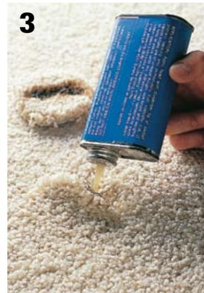
**3 Press the patch into place.** Make sure the direction of the nap or pattern matches the existing carpet. To seal the seam and prevent unraveling, apply seam adhesive to the edges of the patch.
