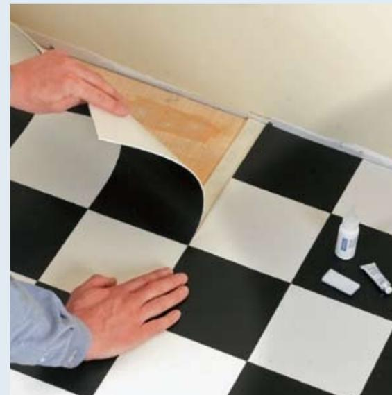
**Center the tape** under the two sides at seam lines. Press one side of the vinyl into place first. Place the second vinyl sheet and press it into place. Use a seam sealer kit to seal the seams.
