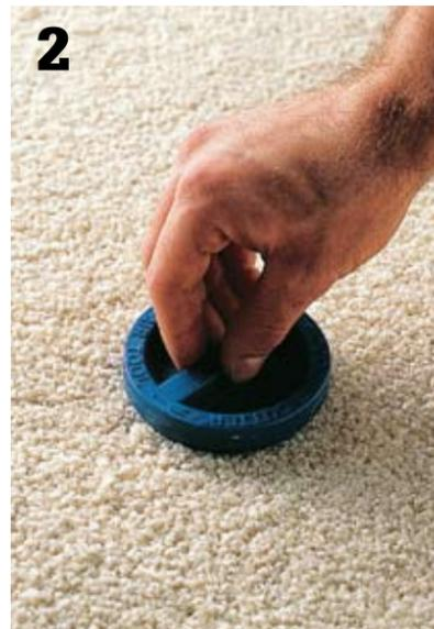
**2 Using the cookie-cutter tool again,** cut a replacement patch from scrap carpeting. Insert double-face carpet tape under the cutout, positioning the tape so it overlaps the patch seams.
